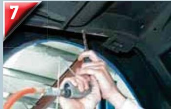
Richard drills two 1/2-inch holes for the TCP 1/2-20x5x3-inch U-bolt that will secure each side. He has scribed each hole location and drilled 1/8-inch pilot holes.
