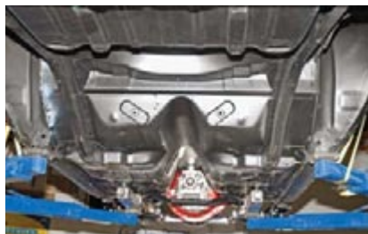
This is how our 99% completed Chassisworks front sub frame looks like from the rear of the car once trial-fitted in place,
