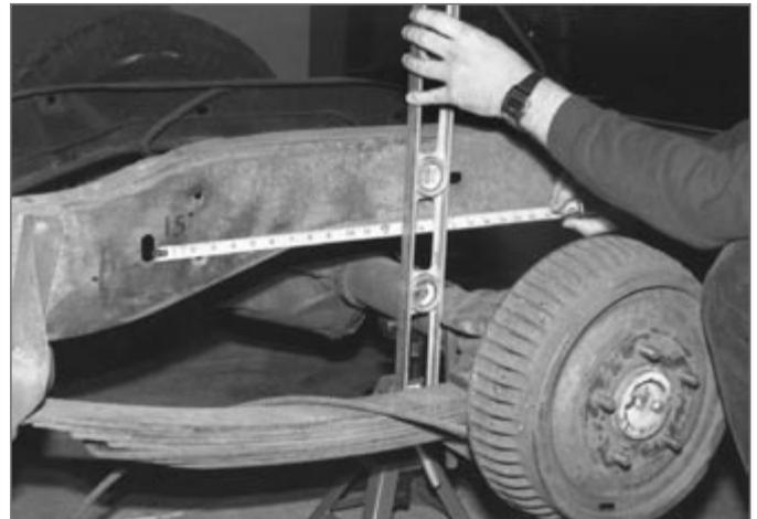
▲ This convenient hole is used as a reference mark on each side of the frame. The distance to the front of the axle housing is recorded to ensure correct housing location upon reassembly.
