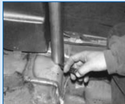
Once the hoop location is finalized, the contour of the floor plate is marked on the ends of the tubing for the trim-to-fit process.
