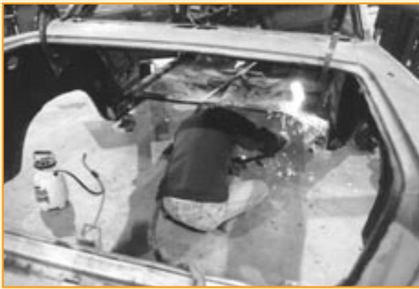
If a torch is used to cut the sheetmetal, be sure to have a water sprayer (visible under the wheel well) on hand to extinguish the flames that will probably result from the undercoating catching fire (water is much less messy than a fire extinguisher in this application).
