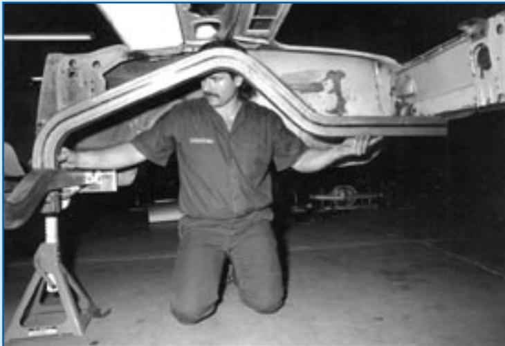
Instruction sheets reveal how to determine the correct frame width for your particular wheel-tire combination. In this case, outside width is 24 inches (note center-line mark on tunnel). Additional measurements are taken between the outside rails and the quarter panels at several points along the subframe, ensuring that the frame is installed perfectly square.
