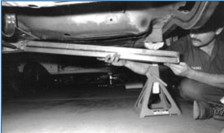
It's easier and more accurate to install the new frame in pieces — using the vehicle to help build it — than to weld it up on a bench, then try to make it fit the car. Chassisworks instructions guide the home builder through every step.
