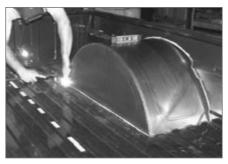
▲ With careful measuring, marking, cutting and welding, a flawless fit is easily attained. This part is a two-man operation, with a cohort underneath the tub holding it in place while the installer tacks it down along the edges.
