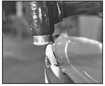
14 A hammer is used to flatten the edge every few inches, joining the two sections. The rest of the protective plastic remains on the tub.
