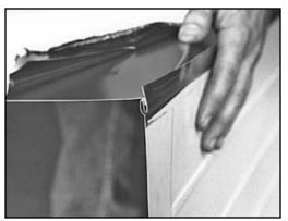
13 Now it's time to assemble the uncut metal tubs. After peeling back the edge of the plastic coating (visible at top left of photos), the two preformed edges are fit together as shown.
