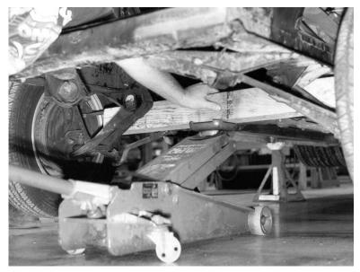
Now you need to prepare to remove the entire front clip. Start by cutting a piece of wood 4x4 to fit under the frame. With the help of a floor jack, it wedges in place in front of the drag link/tie rod assembly and behind the lower suspension control arms.
