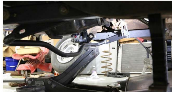
The sway bar is a bit of a pain as well, the two front mounts were installed with bolts, and then we had to use a jack to push the bar into place.
